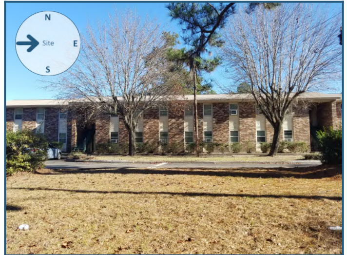
View of site from the west
