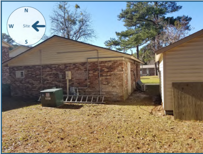
View of site from the east
