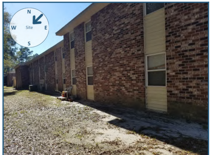
View of site from the northeast
